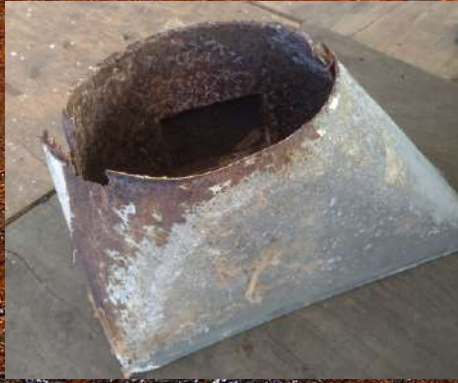
Switchboard Room Deck 13 STBD FZ 2
