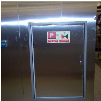
Stainless Steel Recess Door at the Galley area
